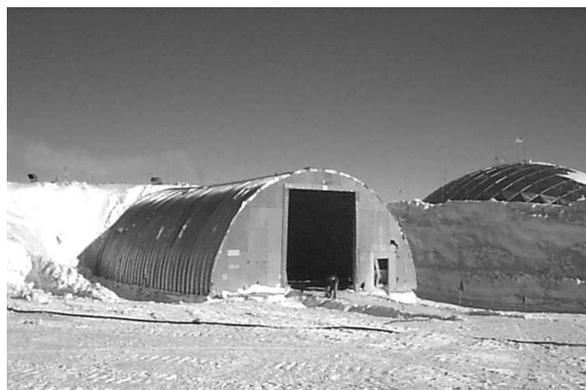
The arc for a *Wonder Building* can be a full semicircle or less than a semicircle. It cannot be more than a semi-circle. The “span” of the building is the total width from one side of the arch to the other.
